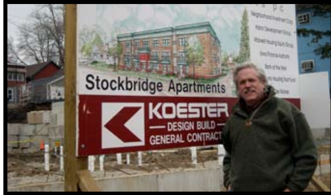
Jack Hatch stands in front of the Stockbridge Apartments construction site.
