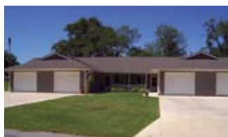
Eastside Townhomes, L.L.C. Oswego, KS 8 units Senior KEF II, L.P.
