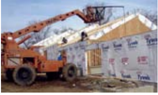
Fontenelle Cottages Limited Partnership Omaha, NE 12 units Senior NF XIII, L.P.
