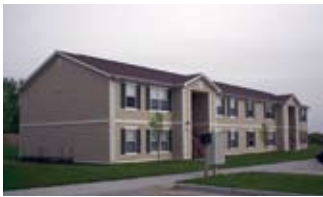
Auburn Housing Partners L.P. Auburn, NE 16 units Multifamily EFN VII, L.P.
