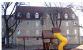
MDI Limited Partnership #104 Winfield, KS 12 units Multifamily KEF V, L.P.
