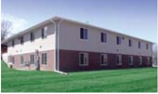
The Center Apartments, LLC Sioux City, IA 22 units Transitional EFN VIII, L.P.
