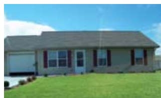
Six Units, L.P. Manhattan, KS 6 units Multifamily KEF III, L.P.
