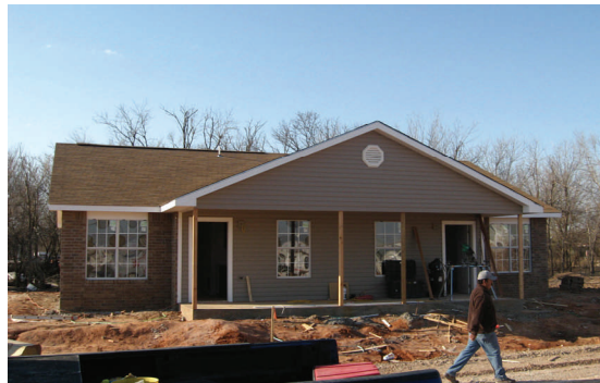
Woodson Park Apartments, OEF II, in El Reno, OK. nears completion.
