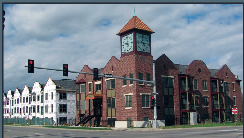
A look at the completed MLK Brickstone Development, LP (IF V, L.P.) and in-progress MLK Brickstone II, LP (IF VI, L.P.). Together the two projects will provide 48 multifamily units for the community of Des Moines, Iowa.
